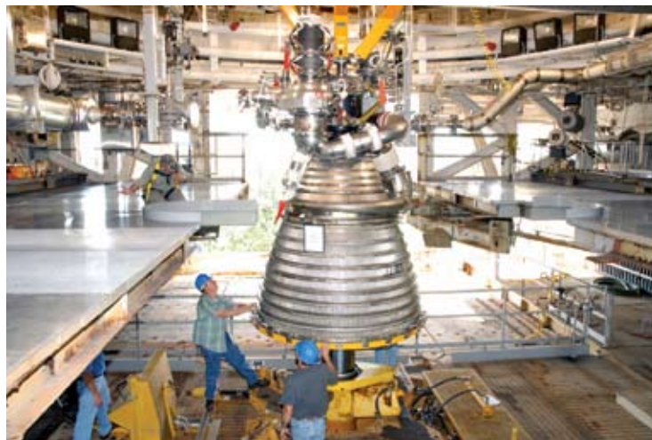
Core components of the J-2X engine for NASA's Constellation program being installed on the A-1 Test Stand at NASA's John C. Stennis Space Center. Tests simulated inlet and outlet conditions that would be present on the turbomachinery during a full-up engine hot-fire test.
