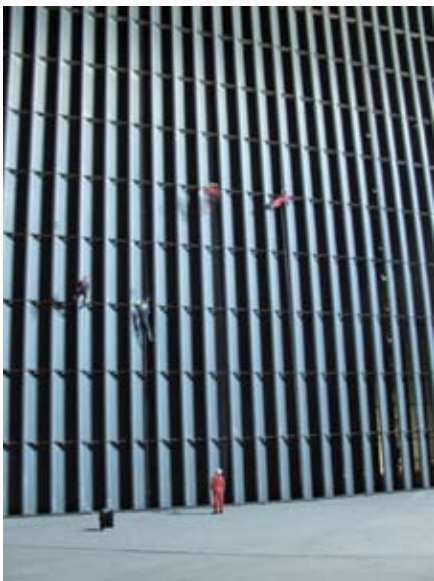
RAT crews inspecting vane set number eight.
