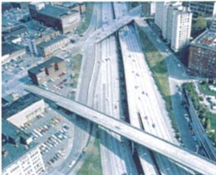
The Convention Center site prior to construction...
