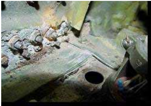
KC-135E Engine Strut Corrosion
