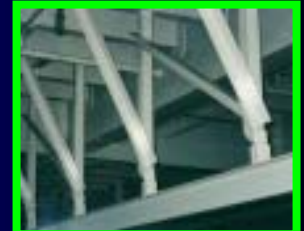
Well-Deck Overhead with specialty coating
