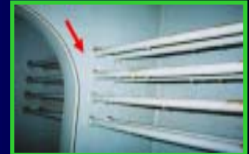
USS Ogden new technology tank coatings after 6 years
