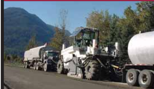
Foamed asphalt repaving
