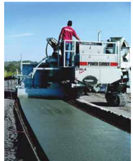
The Power Curber 5700-SUPER-B can pour a sidewalk up to 6 ft (1.8 m) wide in the offset position.
