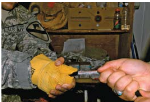
A fiber-optic cable is pulled apart prior to being repaired at a U.S. Army installation in Baghdad, Iraq.
